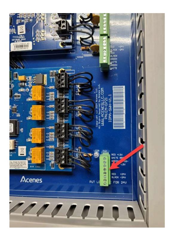
The 8 conductor wire from each door's iDMA has a dedicated connector to wire into. This provides for clean wiring using Panduit wire management.
